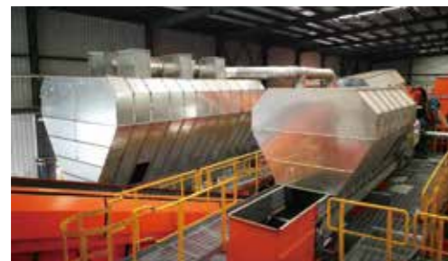
Ghana waste sorting and treating project successfully negotiation. (2000Tons per day)
