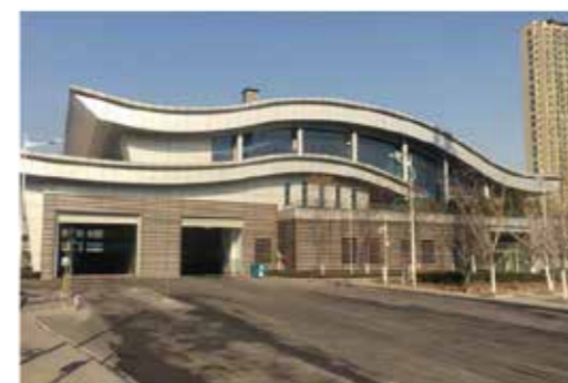
Structure appearance of project
