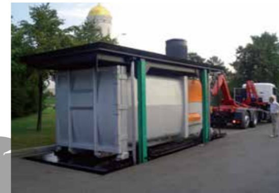
Underground waste equipment in Turkey
